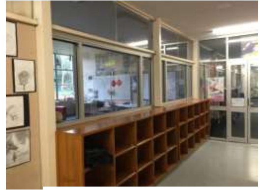
Windows added to Koonga classrooms have increased light and the work spaces available for learning.
